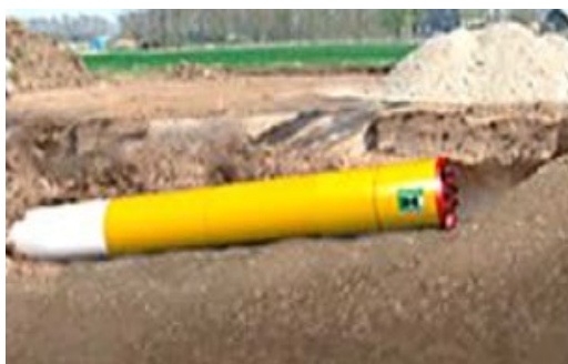
Plate 3.5: MTMB machine at exit location
