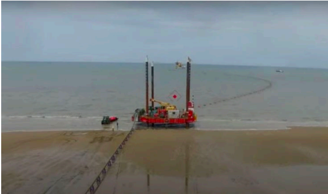
Plate 3.7: Example intermediate pulling platform barge
