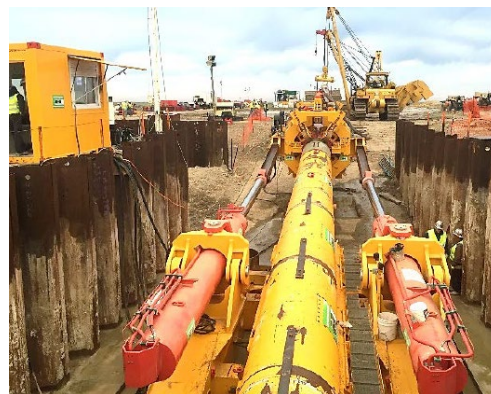
Plate 3.4: Direct pipe thruster equipment at the landfall compound
